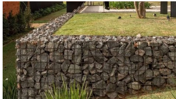
Retaining walls for private gardens with gabions.
